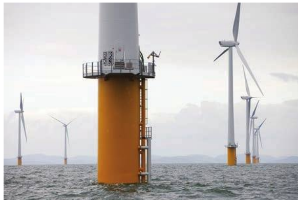
Wind turbines in the Solway Firth on the west coast of the UK. The submerged steel and steel in the water's splash zone must be protected to prevent corrosion.
