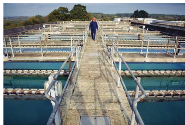
Rapid gravity filter tanks at the River Itchen water treatment works in Southampton, UK. Each tank contains a gravel base and a bed of granular activated carbon.
