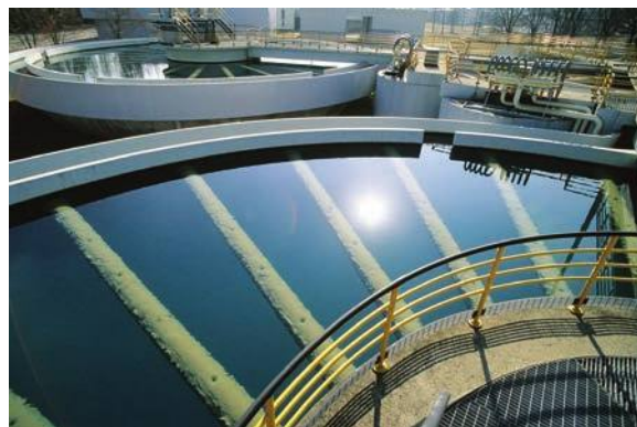
Flocculation and settling stage for purifying drinking water at a waterworks operated by SMAT, the metropolitan water company of Turin, Italy.
