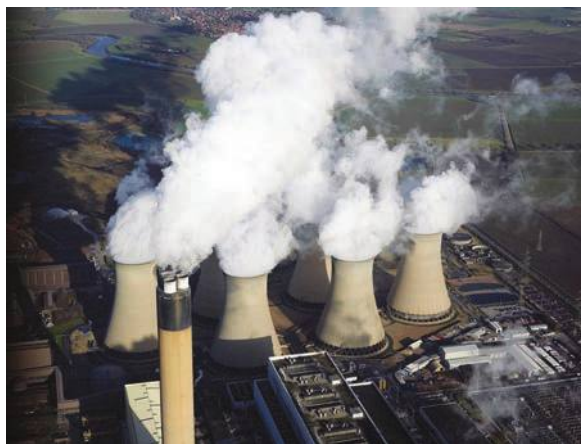
The Drax coal-fired power station in the UK uses desulfurization systems, installed between 1993 and 1996.
