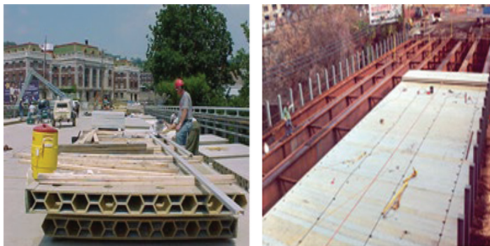
FIGURE 1.13 FRP bridge deck replacement (Market Street Bridge, Wheeling, WV).
