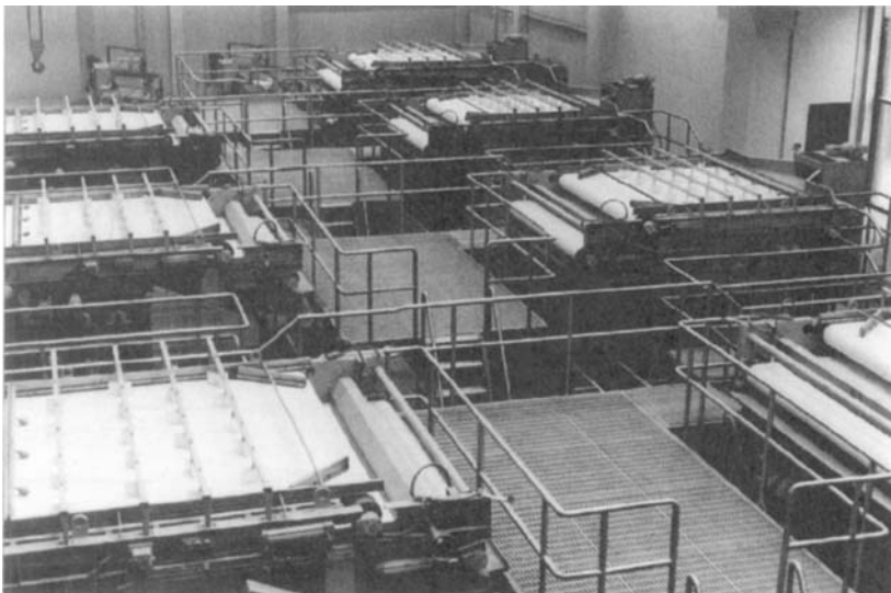
Figure 14.39. Belt presses installed in a municipal sewage treatment plant. (Enviroquip, Inc.)
