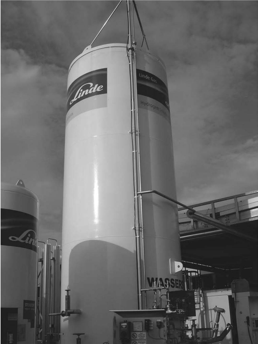
**Figure 1.8** (a) Reservoir tank and (b) conditioning container at the HyCentA Graz.
