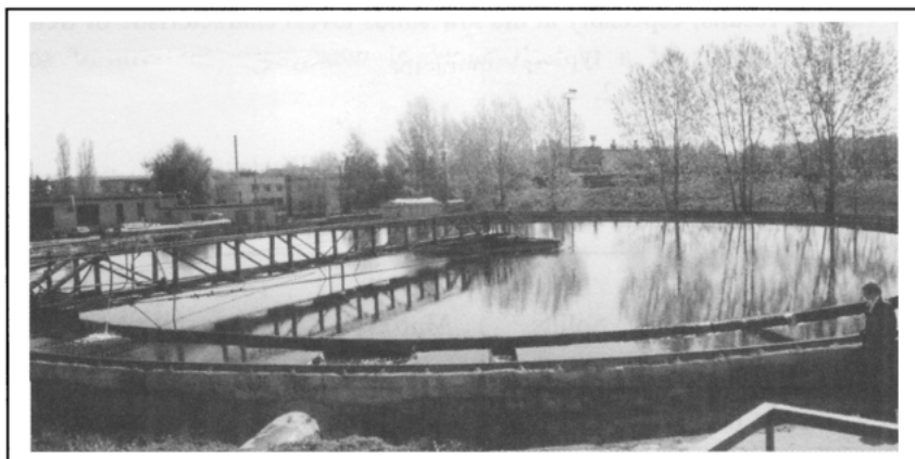
Figure 44. Clarifier in operation in a wastewater treatment plant at the Avtovaz auto-making plant in Russia.
